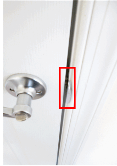
The door to the front right upstairs bedroom would not properly latch.
