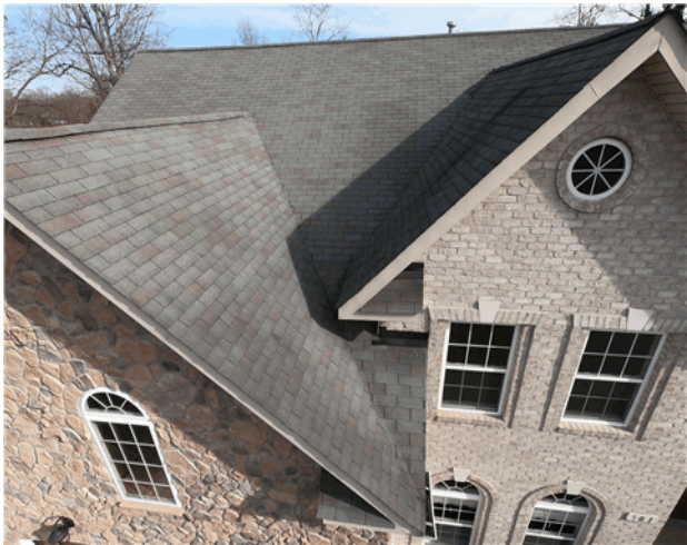
There were several missing shingles at the back of the home (left side of home).
