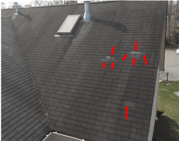
There were several missing shingles at the back of the home (left side of home).
