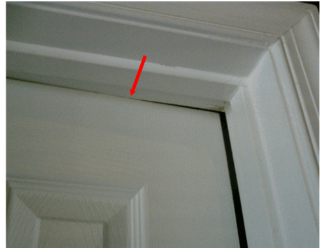
The left closet door in the master bedroom sticks at the door-frame.
