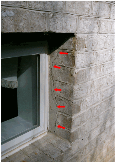
A minor crack in the brick was observed by the front basement window on the right side of the home.
