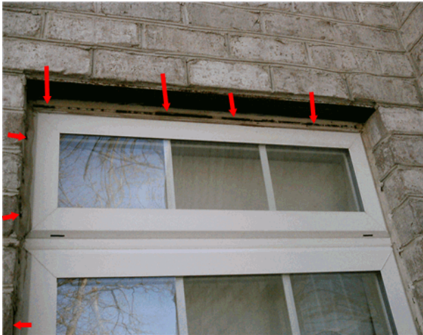
It is important to caulk any cracks / seems in window framing to avoid moisture issues.
