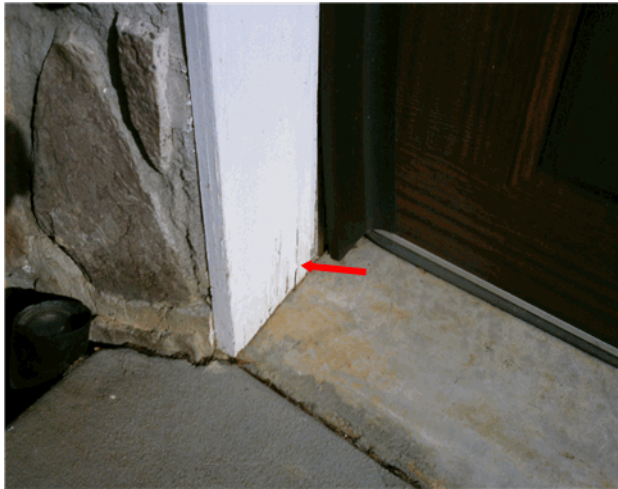
Recommend painting wood door frames that are weathered to help prolong the life of the wood.
