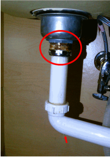
The drainpipes under the left sink were actively leaking at time of inspection.
