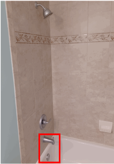
Water came out of tub spout while shower was on in upstairs hallway bath. (Diverter issue)
