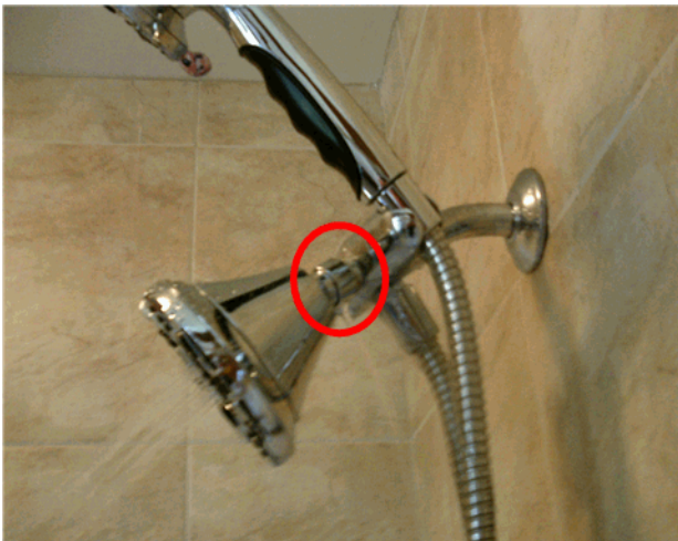
Water squirted out at the threads of the shower head in the master bathroom shower.
