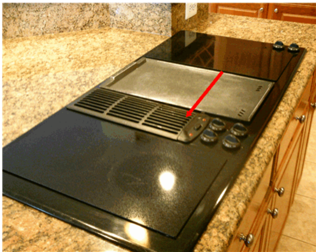
Exhaust fan built into cooktop.
