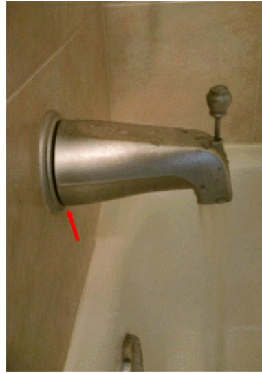
There was also water coming out of the back of the tub spout in the upstairs hallway bathroom.
