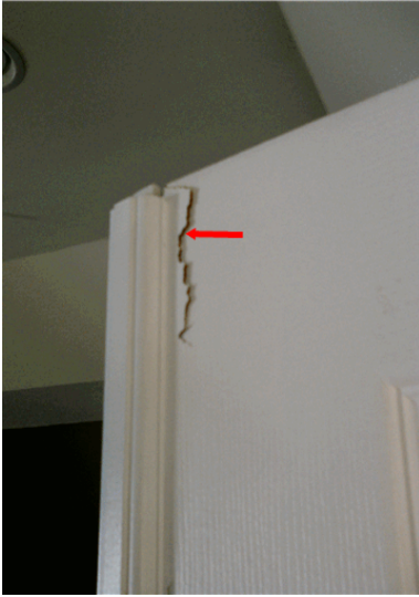
The master bedroom door was damaged at the top by the lock.
