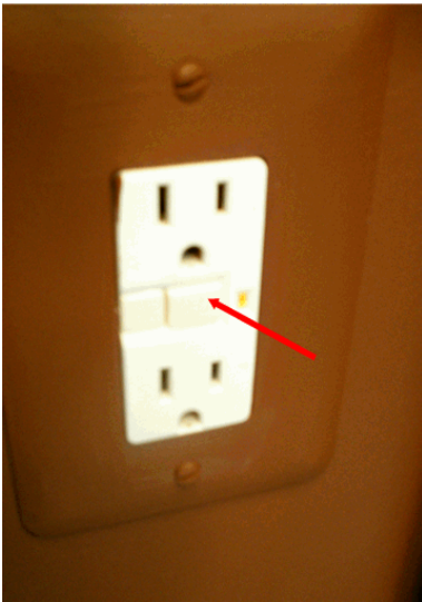
Electrical outlets in all baths are tied into GFIC in master bath. (Push here to reset)
