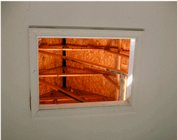
The attic access in the garage was missing the panel / board at time of inspection.
