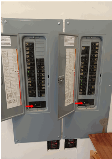
Main electrical shut-offs. (Shuts off power to entire home when both are off)
