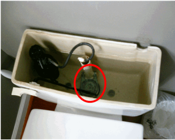
The toilet in the half-bath on the main level had a sticky flapper.
