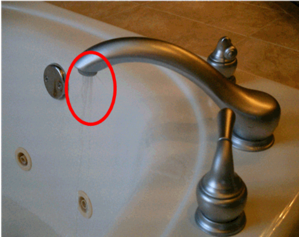
The whirlpool tub took way longer than it should (2 hours) to fill up past the level of the jets.
