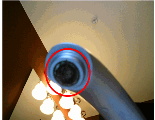
The aerator for the whirlpool appeared to be clogged, blocking proper water flow.
