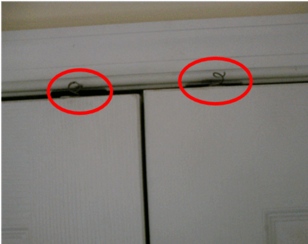
The locks at the top of the closet doors in the front right upstairs bedroom were damaged.
