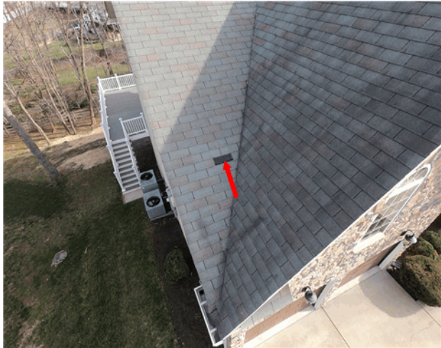
There was one missing shingle at the front of the home.
