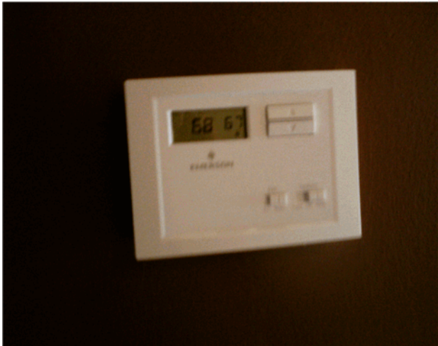
Thermostat on second level controls temperature on the top level.
