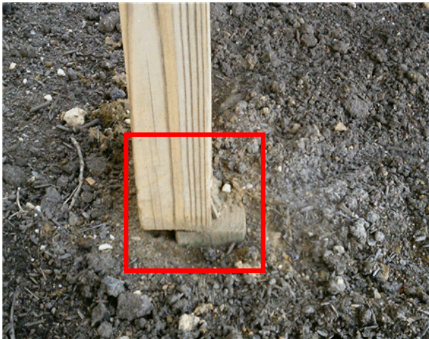
The right support post for the deck stairs appeared to have been cut. (Safety issue)
