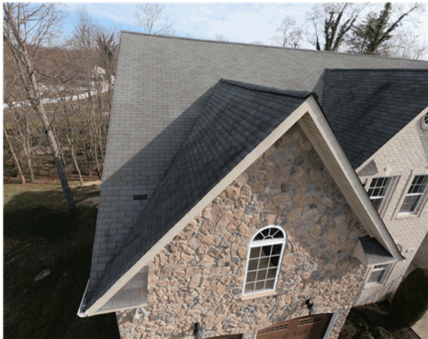
There was one missing shingle at the front of the home.
