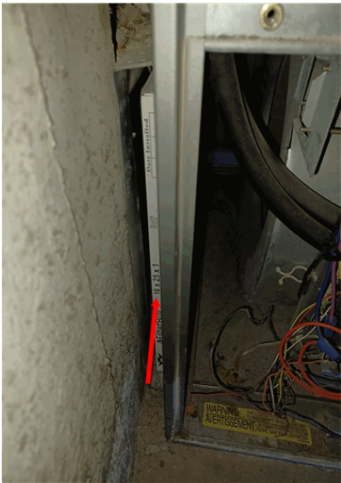
16"x25"x1" air filter goes here. (Unit in Basement) (Replace every 30-90 days)
