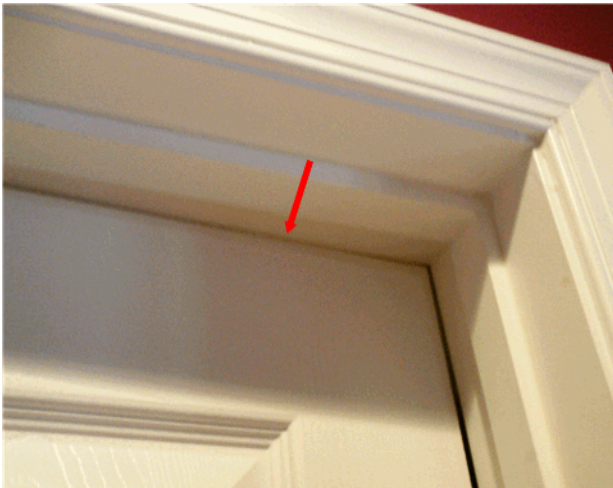
The door to the utility room in the basement sticks at the door-frame.
