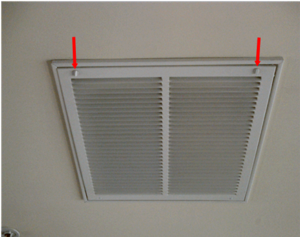
16"x16"x1" air filter goes here. (1 of 2 upstairs) (Replace every 30-90 days)
