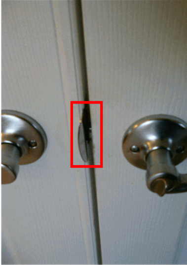
The master bathroom door did not properly latch at time of inspection.
