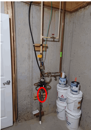
Main water shut-off. (Shuts off water to entire home)
