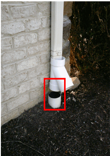
The down spout at the front left corner did not extend into the sub-surface drainage system.
