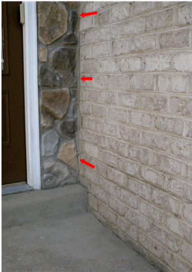
Recommend re-sealing where the stone veneer wall meets the brick on both sides of front entrance.
