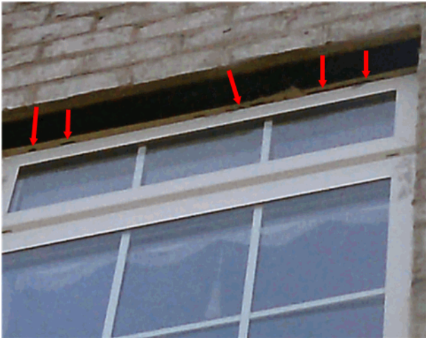
Some of the windows are in need of re-caulking around the exterior of them.
