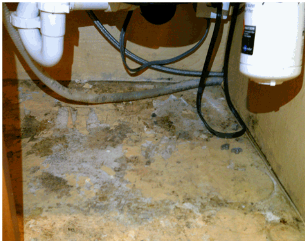
The cabinet under the kitchen sinks had water damage at the bottom.
