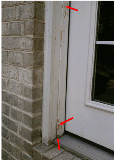
Recommend painting wood door frames that are weathered to help prolong the life of the wood.
