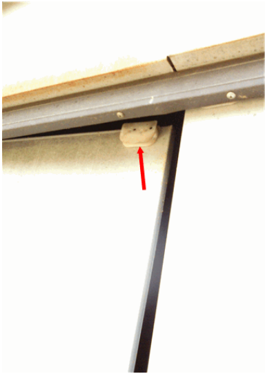
The left shed door was off track at time of inspection. Recommend repair / adjustment.
